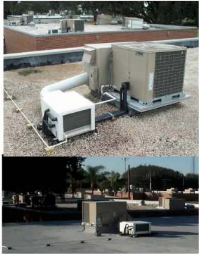
An Average 38% Improvement Over the Manufacturer's Original Rated EER
